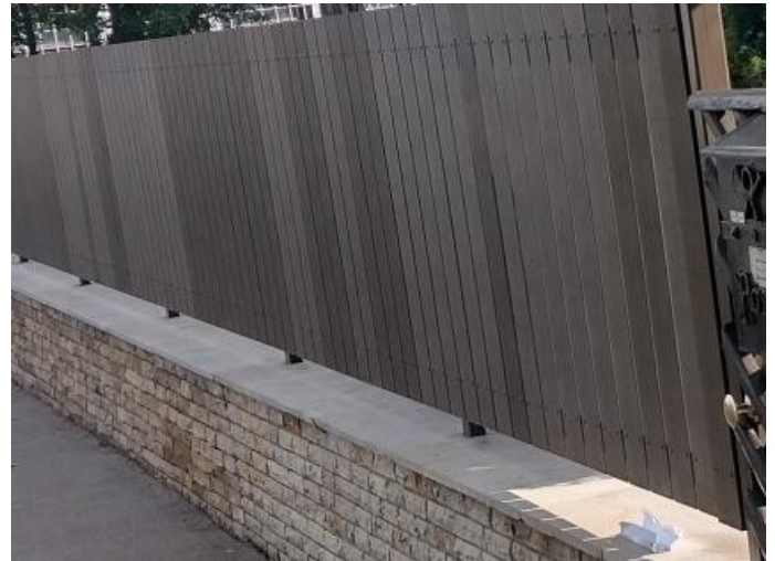
Fig. 11 Colour difference when the fence panels are not installed in the same direction
